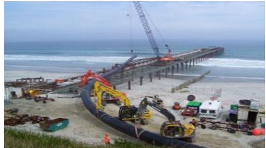
Christchurch Ocean Outfall
